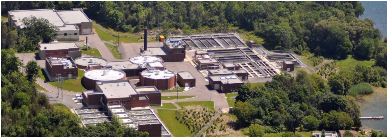
Figure 4 - Ravensview Wastewater Treatment Facility, Kingston, Ontario*
